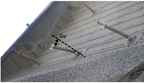
Figure 5. Inspection of the nails after the test.
