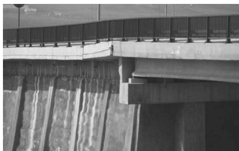
Figure 4 Zone between embankment - bridge.
