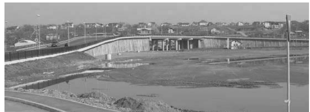
Figure 1 General view of the embankment
