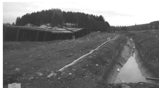
Figure 1 Test site after the failure. Instrumented area is between the containers and the ditch. Loading structure has overturned and the slip surface is protruding from the ditch.
