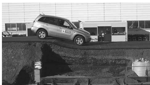
Photograph 4. Trial embankment after testing of 550mm differential settlement. (Confined-Reinforced Earth tested in Ibaraki, Japan, 2011)
