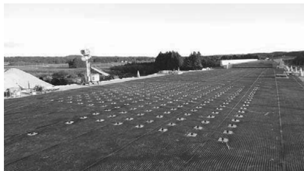
Photograph 3. Application of Confined-Reinforced Earth for actual highway embankment in Joban Highway, Fukushima, Japan, 2011.
