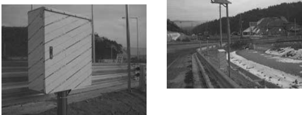
Figure 3. Placement of measuring instrument on the compacted roadbed materials
