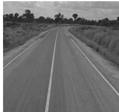
Figure 4. Finished road at trial section
