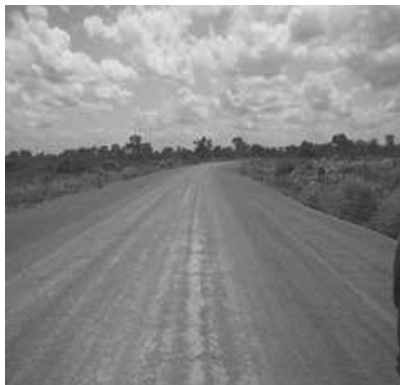
Figure 2. Compacted shale at trial section
