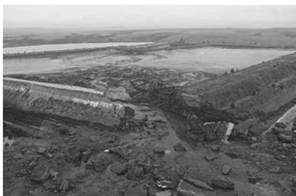
Figure 1. Ajkai Timfoldgyar dam failure.
