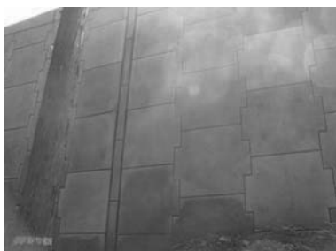
Photo 8. No damage Section of Anti-frost heaving (After the 2011 Tohoku Earthquake)
