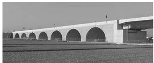
Figure 1. Multi-arch culverts embankment
