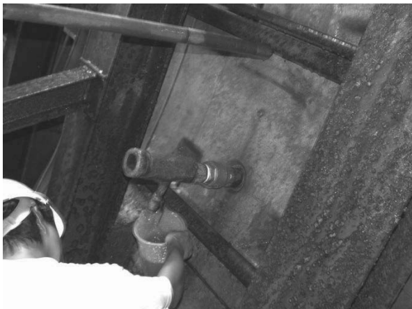
Figure 6. Water-leak test before cross passage excavation.
