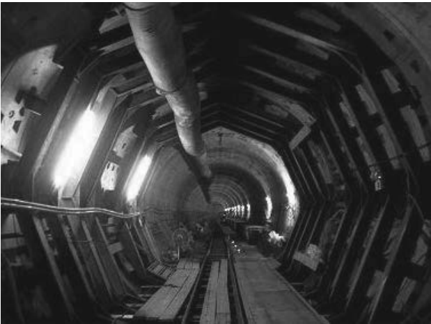
Figure 9. Octagonal steel-beam reinforcement inside tunnel.
