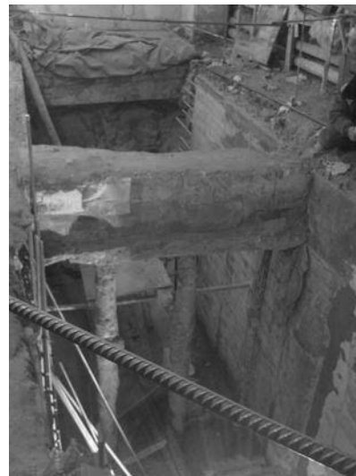
Figure 8. 4.5 m deep service duct
