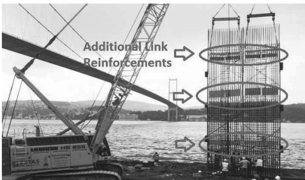
Figure 11. Additional Link Reinforcements on the Slab Elevations
