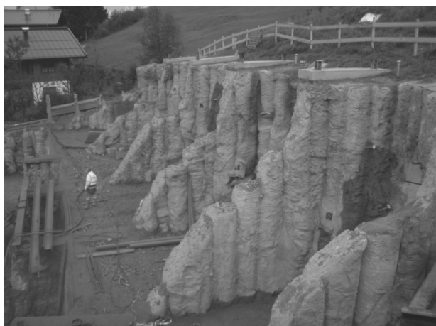
Figure 6. View of excavated MIP-walls
