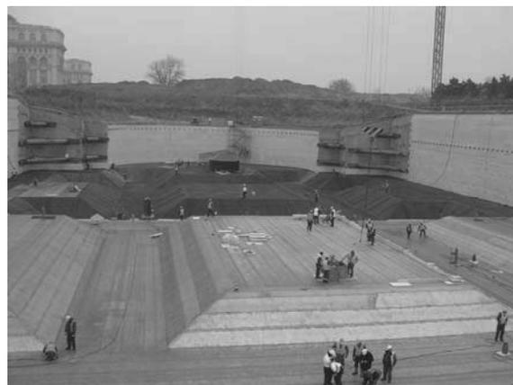
Figure 9. Lead waterproofing
