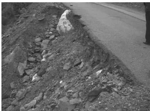
Figure 1. Photo of local slope failures
