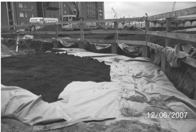
Figure 5: Placing of expanded clay
