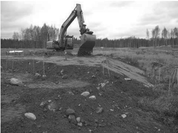
Figure 5 Construction up to height 1.5 m for embankment 1.
