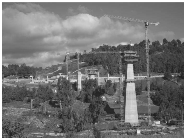
Figure 15. Status of P4 construction December 2012
