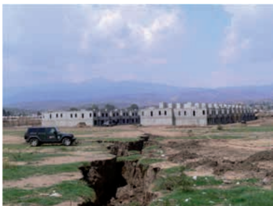
Figure 4. A dramatic example of soil fracturing in a site near Mexico City
