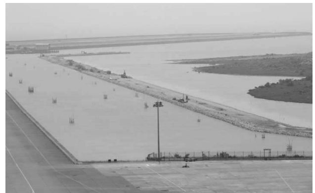
Figure 13. The Completed Stone Column Seawall
