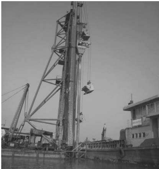
Figure 11. Stone Column Plant for Wet Bottom Feed installation
