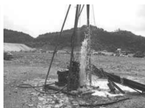
Figure 10. Ejection of leachate/gas
