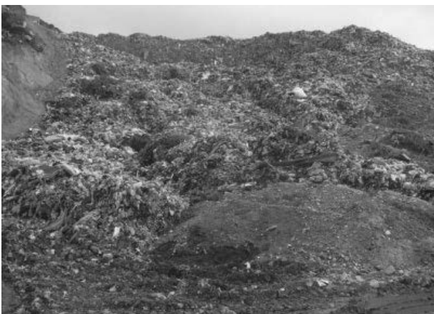
Figure 3. Waste slide view from the access bench located at the toe of the slide.
