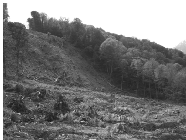
Fig. 6. Ski-jump site at the beginning of construction operations
