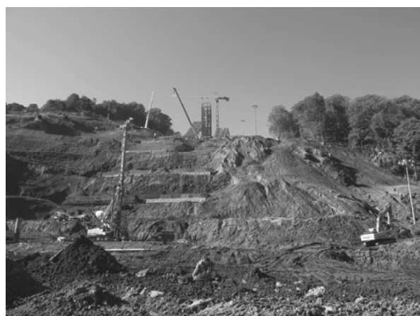
Fig. 7. The same terrain during footing erection
