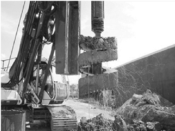
Figure 3. A twin-flight auger used for the East London trial.
