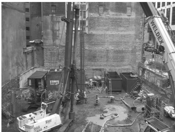
Figure 1. The small site in Glasgow where a polymer fluid was used.
