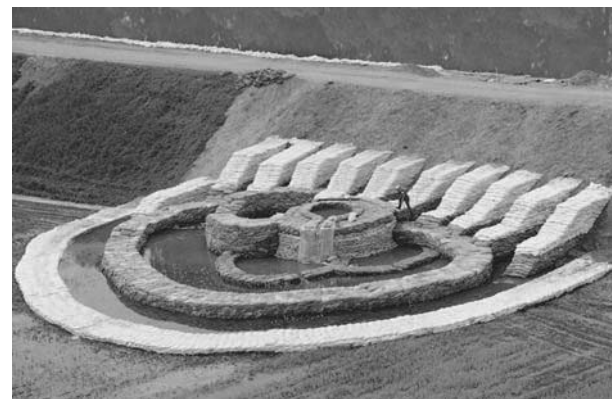
Figure 5. The giant piping at Tiszhasa/Hungary in 2000 and stabilizing measures (Nagy, 2011): Reduction of hydraulic gradient and lateral support of dyke slope.
