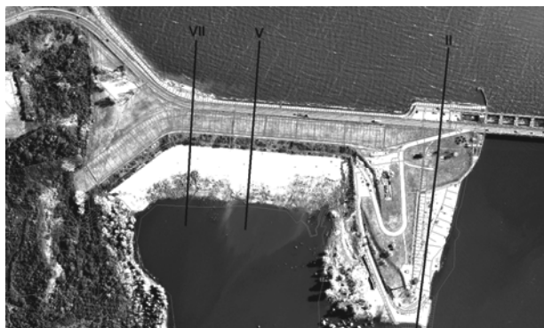
Drawing 1 Earth dam location plan showing the orientation of cross-section taken for calculations
