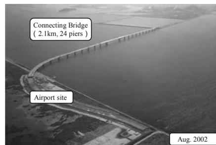
Figure 1. Overview of connecting bridge under construction
