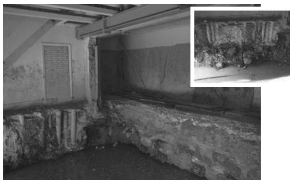
Figure 1. Indoor wet excavation.
