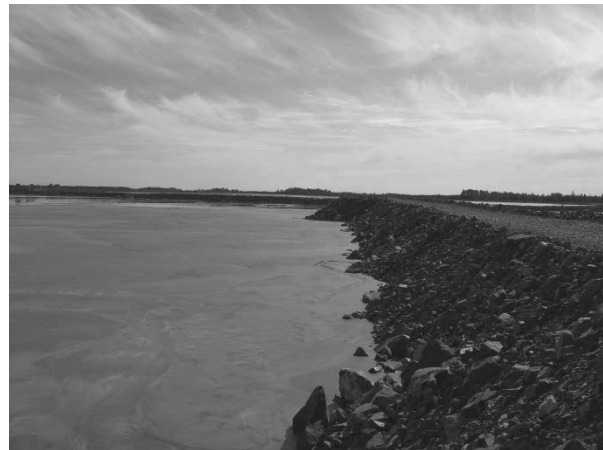
Figure 3. A waste rock inclusion in a tailings impoundment at a mine in western Quebec.
