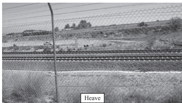
Figure 5. Bulge of the surface above the caisson. Observe the reduced thickness of the ballast layer
