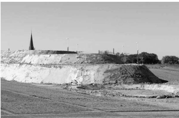
Figure 1. Landscaping with stabilized soil.
