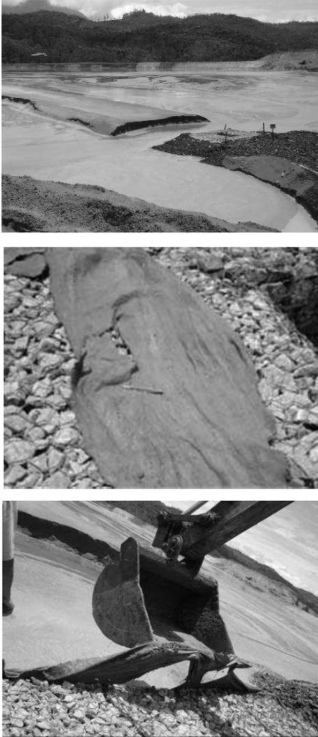
Figure 2: Exhumation of the geotextile sample.
