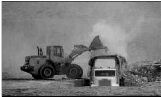
Figure 2. Front-end loader dumping soil into a haul truck with no dust control method implemented (Maricopa County 2009).
