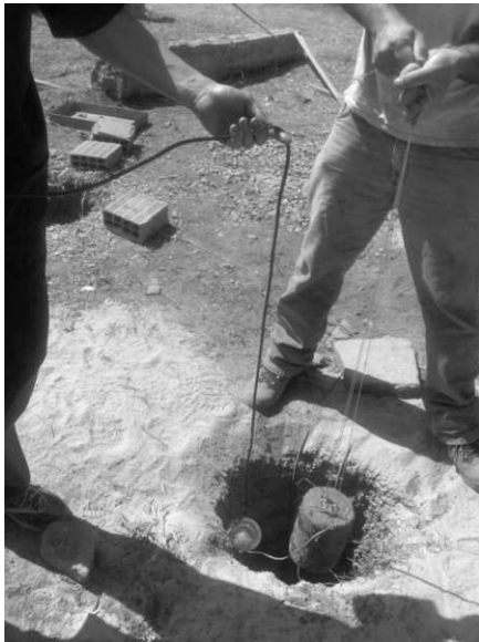
Figure 4. Placement of a strain gauge in the column.
