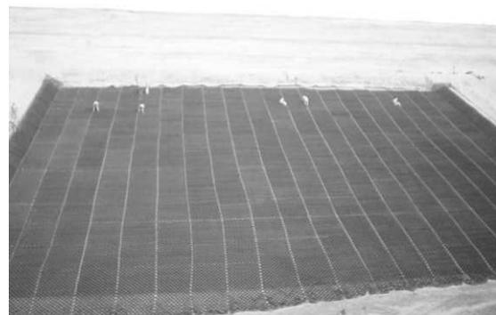
Figure 7. Geocells expansion/ Geotextile placed.
