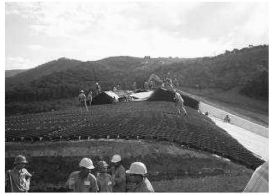
Figure 12. Detail of the geocells flexibility.
