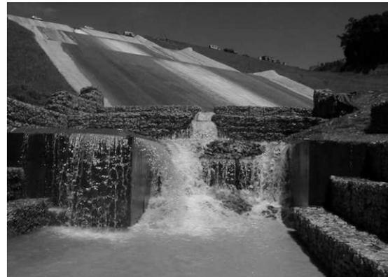
Figure 14. Final dissipation basin.
