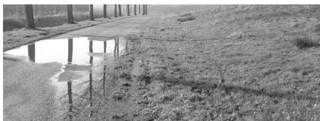
Figure 5: Occurrence of puddle at toe inner slope
