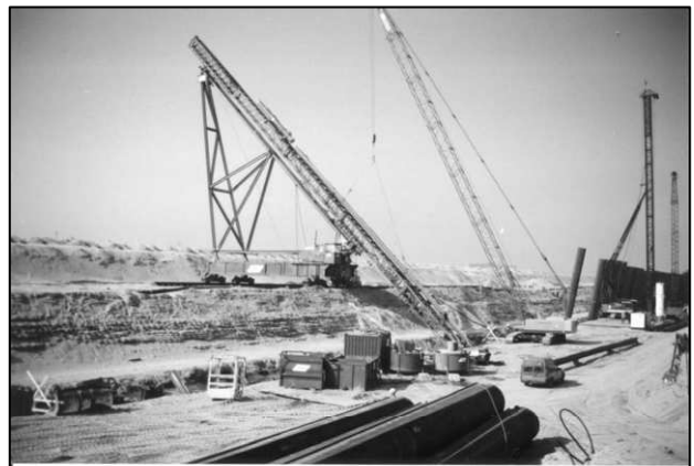
Figure 4 Pile Installation
