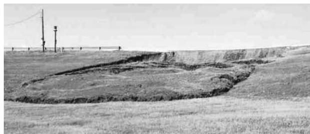
Figure 2. A typical surficial failure at Joe Pool Dam.
