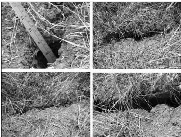
Figure 6. Desiccation cracks along construction joint.
