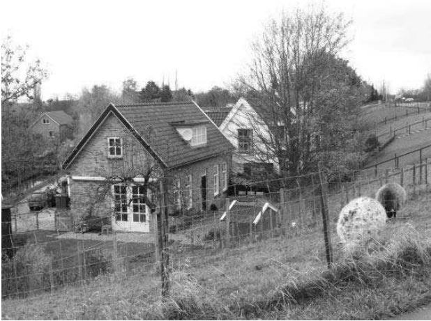
Figure 2. Dike at the reinforcement project Bergambacht - Schoonhoven
