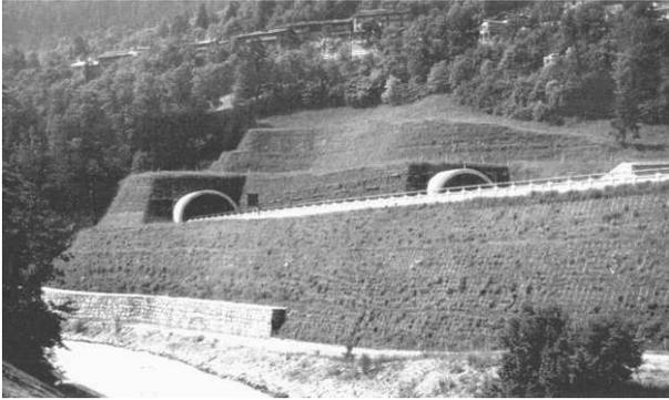
Figure 1. A sample of integration of buried precast arches and inclined reinforced earth structures.
