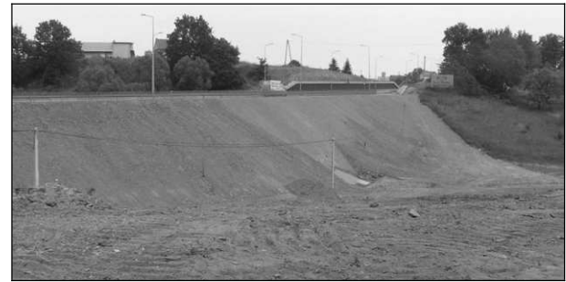
Pic. 10 The view of road after stabilization of the landslide
