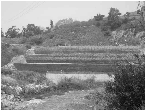
Figure 2. Phase of the stabilization project construction.
