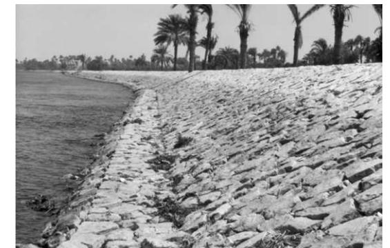
Figure 7. River bank protection two years after construction.
