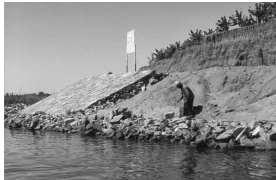
Figure 6. Partly completed river bank protection.
