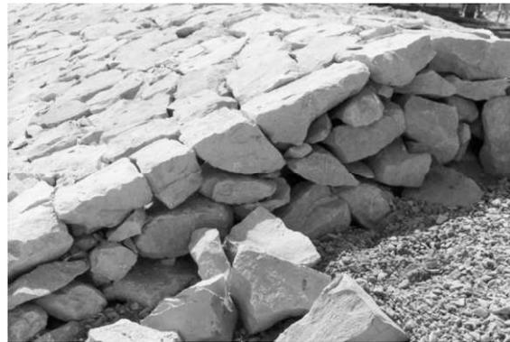
Figure 5. Detail of the stone revetment atop gravel filter layer.
