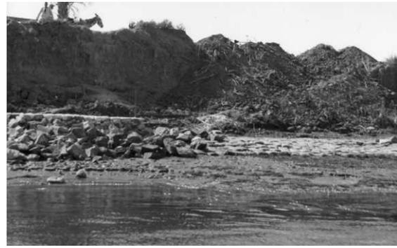
Figure 4. Stone toe atop sandbags under construction.
