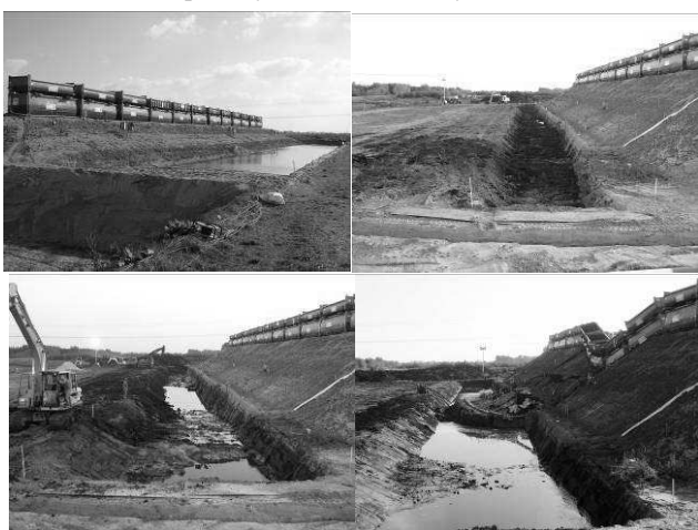
Figure 8. a) River side of the dike, b) Inner side of the dike during excavation of the ditch, c) Inner side of the dike after excavation of the ditch, d) Failure
