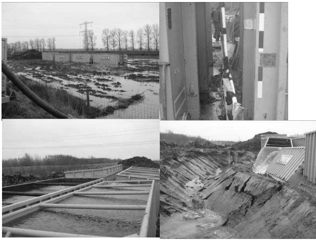
Figure 4. a) Overview preliminary test b) Measurement row at the centre of the container row c) Filling of the containers d) Failure
