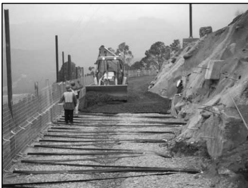
Figure 11. Langeni – synthetic reinforcing strips
