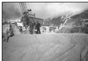
Figure 3. Church Street under construction
