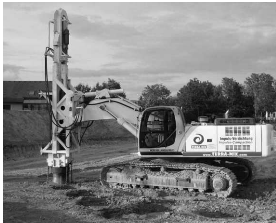
Figure 7: Rapid Impact Compactor (RIC).
