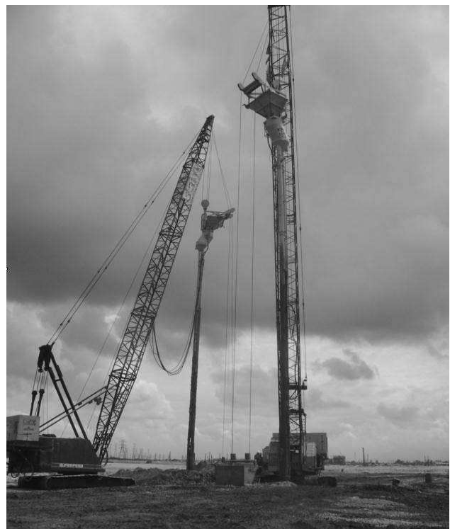
Fig. 5: Installation of stone columns using Alpha-S type vibrator (Keller Grundbau GmbH).
