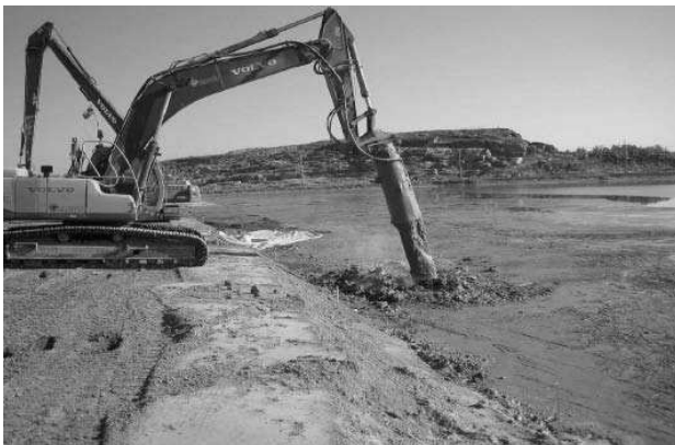
Figure 4. The mass stabilization of dredged TBT -contaminated sediment.
