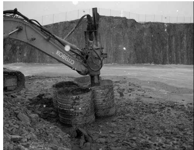
Figure 1. Mass stabilization test in the temporary storage basin of TBT-sediment..
