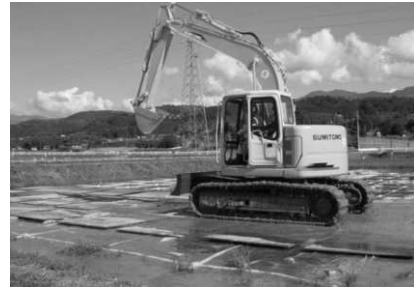
Figure 10. Installation for temporary approach in wet paddy field
