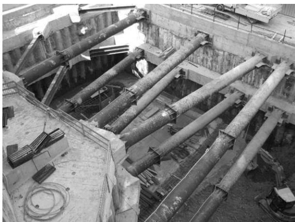
Figure 4. The two levels of struts and the excavation at full depth.
